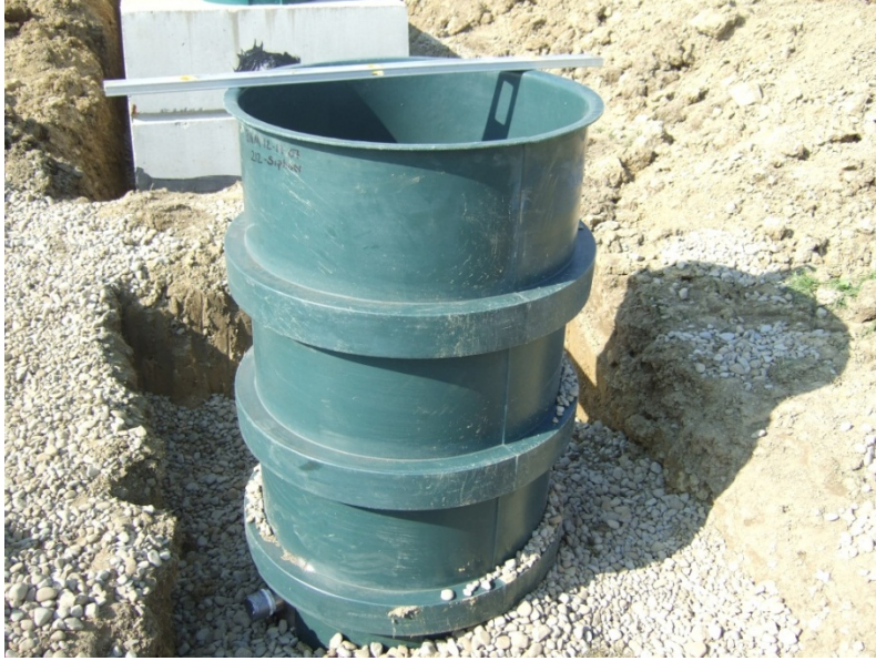
Figure 5. Dosing siphon - external view
